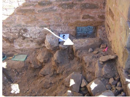
Figure 2. Arrow pointing to rock support for sliding box (inside wall Hospital)
