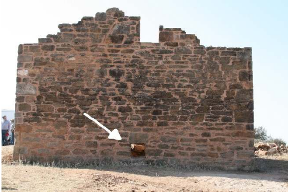
Figure 1. Arrow pointing to square hole in north wall Post Hospital Fort Chadbourne
